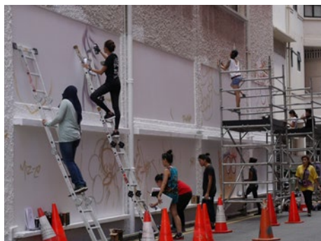
Work in progress / Queen Street, Singapore / 2014
